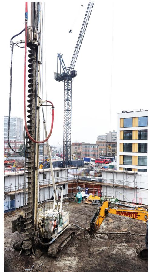
*A Soilmec SF50 was used to carry out the piling works*
