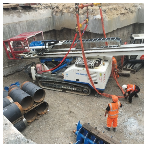
Craning operation for lowering the SM-16 rig into the excavation
