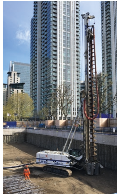
Installation of bearing piles inside basement
