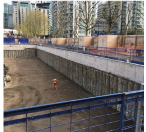
Secant pile wall at Harbour Central
