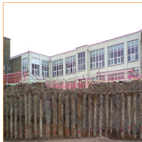
Exposed secant wall
