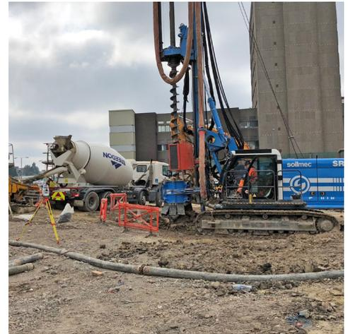
*Soilmec SR-45 installing CFA bearing piles.*
