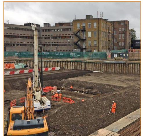
*Soilmec R-210 installing Rotary bearing piles.*
